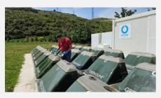
Since April 2025, a comprehensive **monitoring campaign has been underway in Türkiye** to evaluate the pilot system's performance and environmental impact. Weekly sampling at both the inlet and outlet, as well as across all photobioreactor (PBR) lines, includes chemical analyses (PFAS, PAHs, PCBs, phenols, pesticides, heavy metals) conducted by TÜBİTAK MAM's accredited labs.
