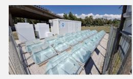
The RHE-MEDiation project has successfully installed its third and **final demonstration site in Taranto**, Italy, **along the Galeso River**. Also this site features the GREEN DUNE® photobioreactor system designed to remove chemical contaminants using algae-based treatment. Fully equipped with CO<sub>2</sub> injection, nutrient dosing, biomass collection, and remote monitoring, the system offers a nature-based, scalable solution to improve water quality.
